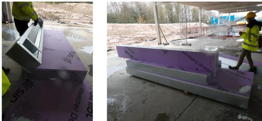
Fig. 3. Pre-assembled lightweight exterior infill wall panels.
