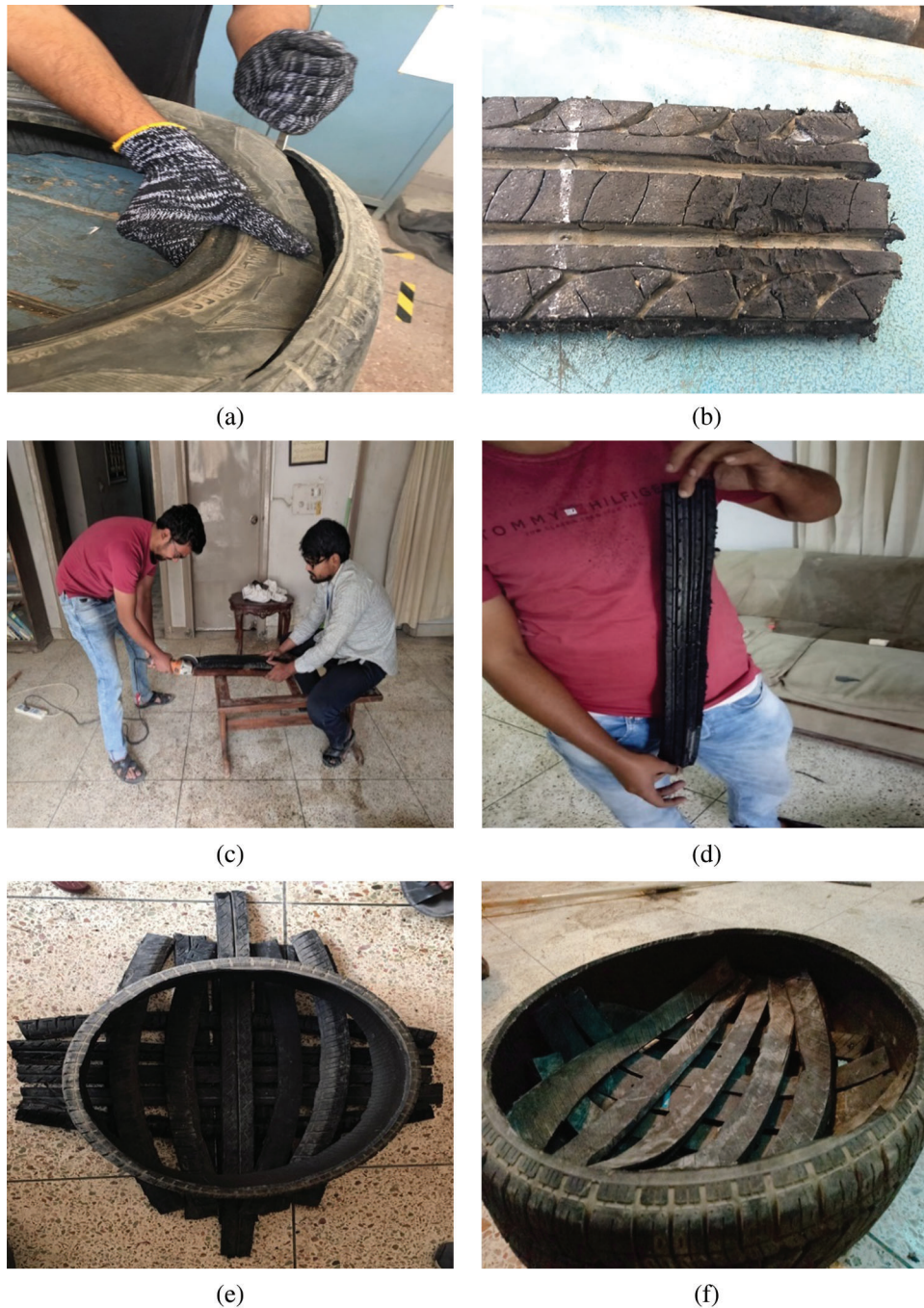
Figure 4: Preparation of rubber strips and rubber mold frame for the casting of a manhole cover (a) Cutting of tire for separating tire tread (b) Tire tread (c) Cutting of tread through a grinder for rubber strips (d) Rubber strip used (e) Rubber tire mold for manhole with rubber strips (f) Orthogonal/Hash orientation of rubber strips in the mold
