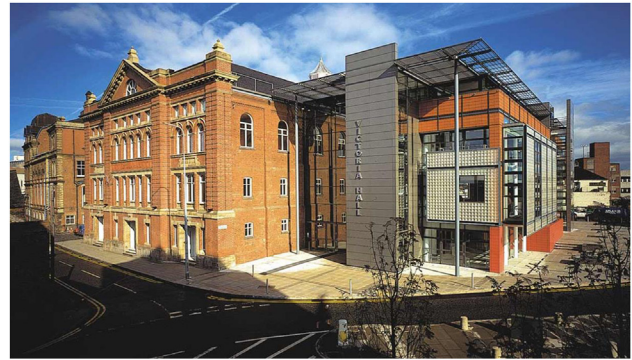
Fig. 4 The recess of the new building facade compared to the historical facade of Victoria Hall in Staffordshire, England. Source: The times.
