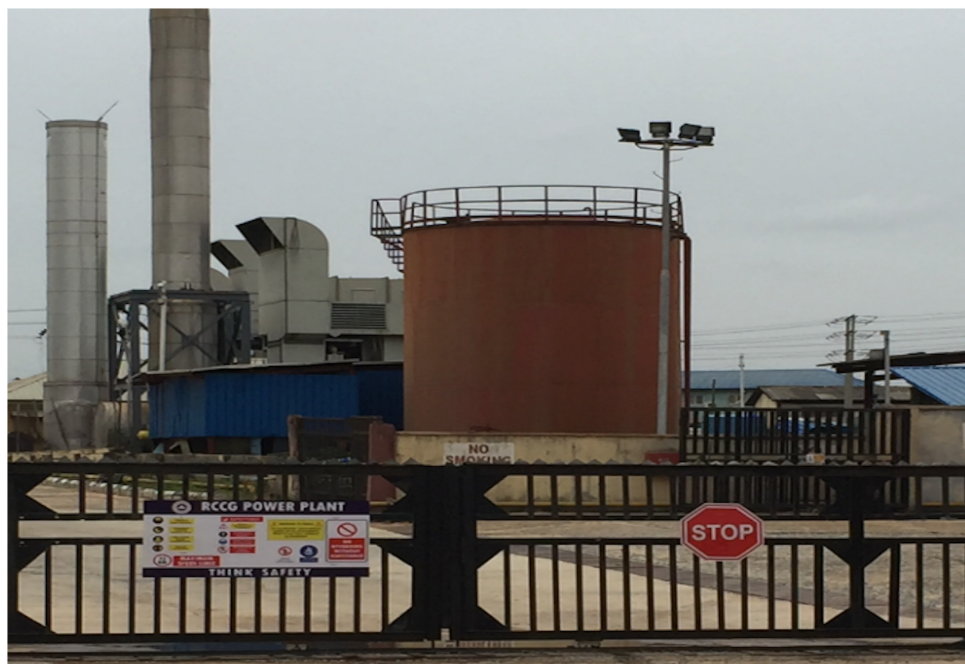
FIGURE 2 The current Redemption City power plant (photo by Gareth Millington, June 2018)
