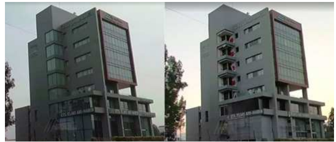
Figure 7 Different damage observed for different glazing orientations at Location 3; before [left] and after [right] the explosion [3]
