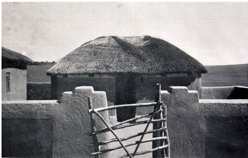
Figure 2. Ndebele homesteads outside of Johannesburg photographed by Betty Spence. Betty Spence, “Native Architecture,” South African Architectural Record (November 1940): 387–91.
