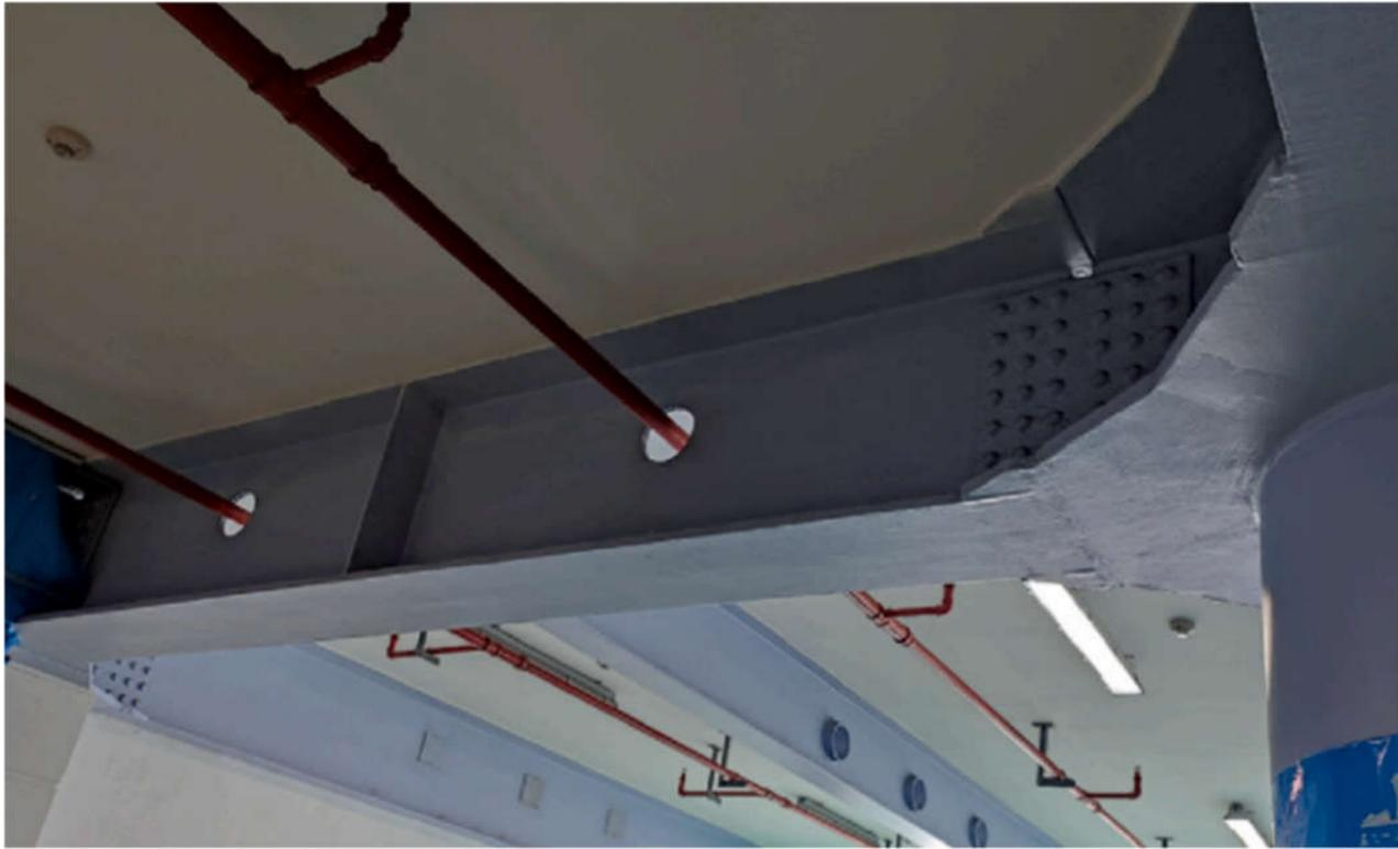
**Fig. 1. Engineering application of perforated plate girders**
