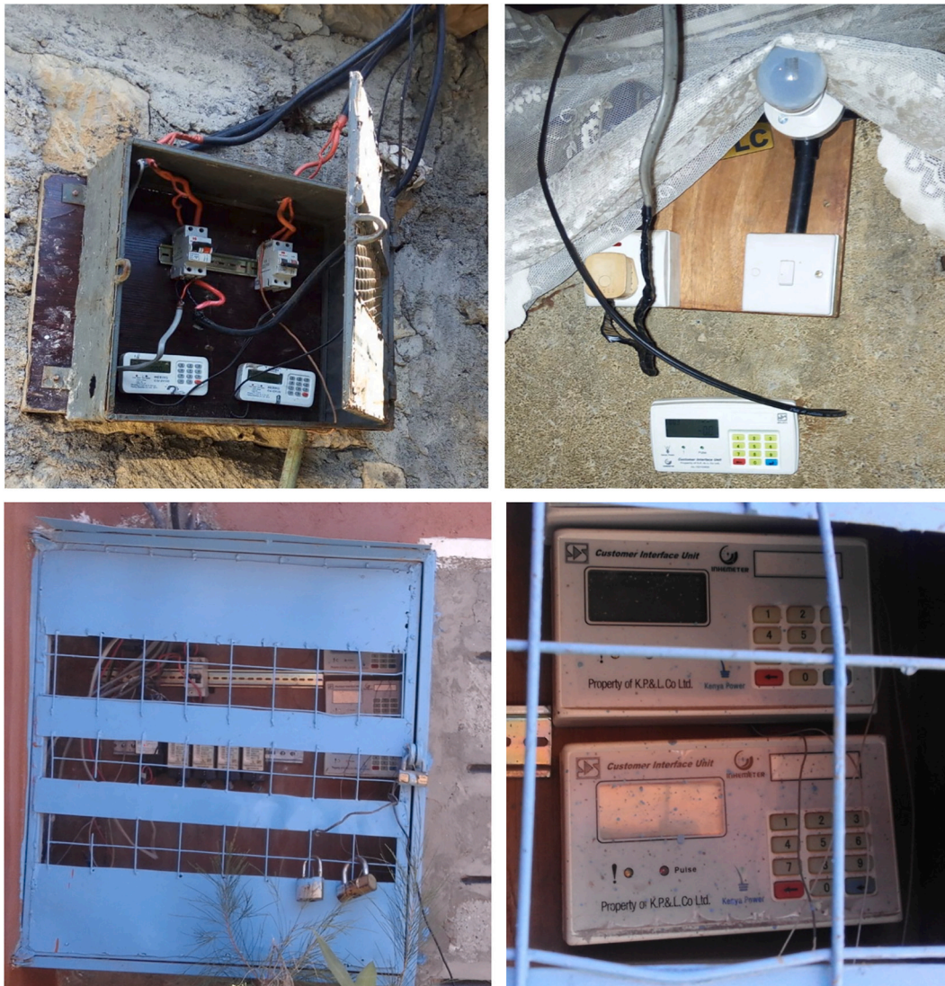
Fig. 1. Outdoor and indoor ready boards and customer interface units. Images by lead author, Kibera, 2016.
