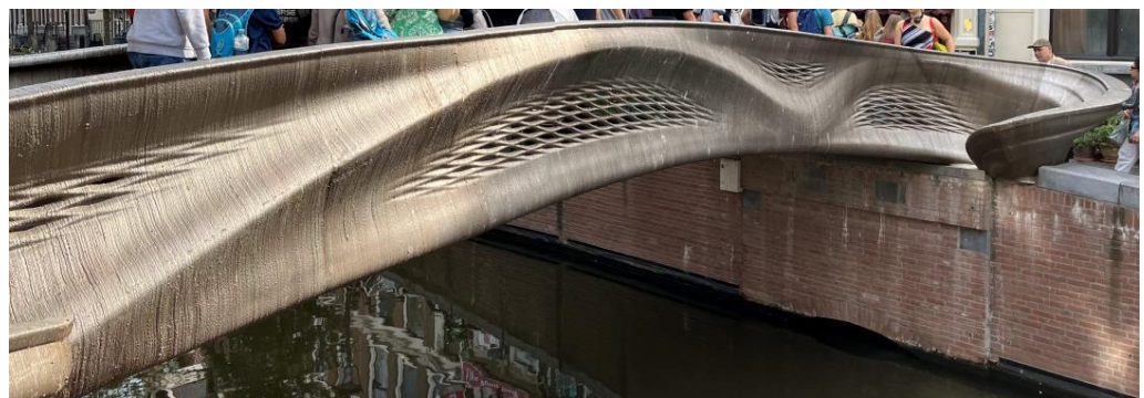
Figure 10. Additively Manufactured Bridge.
