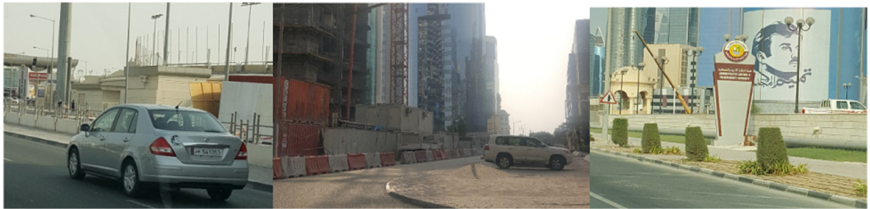
Fig. 17. No Shading Devices on Main Streets (Source: authors).
