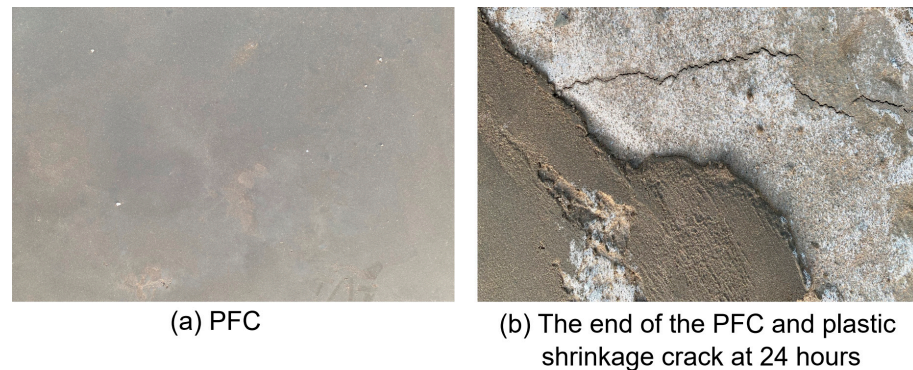
Figure 8. Concrete surface finish after the power floating of in situ large-scale slabs: (a) inner area, and (b) edge of slab.
