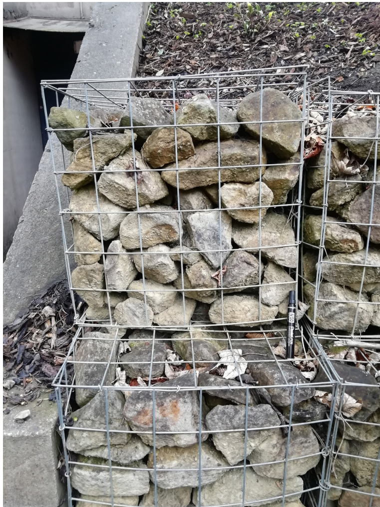
Figure 3. Gabions in use for landscaping. Here filled with blocks derived from Permian age dolostones. The use of such structures to display cobble materials enables the incorporation of such materials into geo-educational structures such as rock trails.
