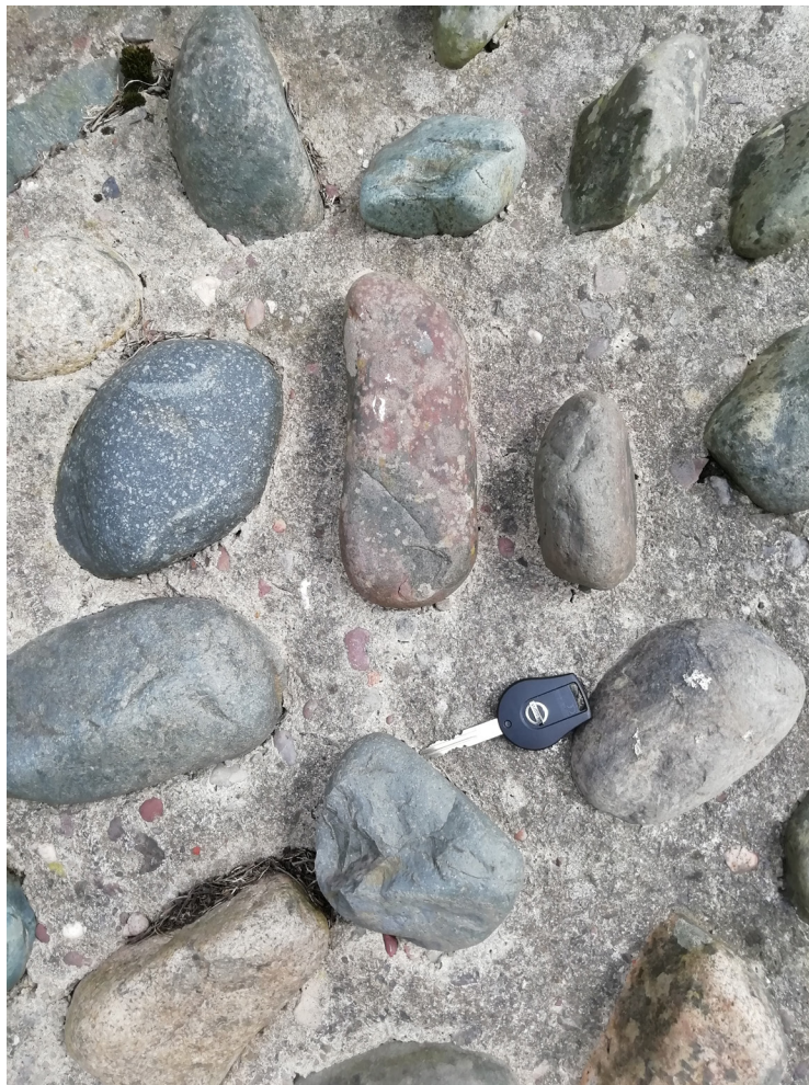
Figure 1. The incorporation of cobbles derived from glacial till into concrete. A common site in post-World War 2 redevelopment sites.
