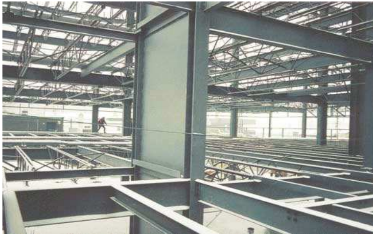
Figure 1. Steel plate shear wall system [25]
