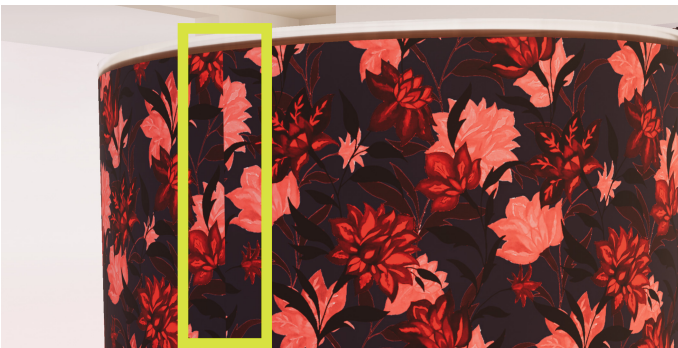
Fig. 3. Incorrect application of pattern caused by non-matching edges
