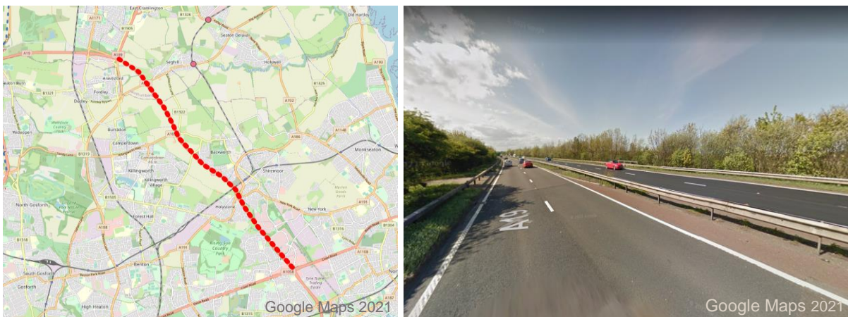
Figure 10: Scheme length, location and the 'street view' of the A19 junction and on-line improvements between Killingworth interchange and coast road/Silverlink interchange, planned for the route upgrade
