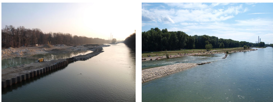
Figure 25. The Isar river (Germany) during (left) and after (right) the hydro-morphological restoration. It is one of the main tributaries of the Danube, sources in the Alps, and crosses the Bavarian capital Munich. Heavy rain events in the Alps in the years of 1999, 2005 and 2013 led to major floods. Today's near-natural landscape raises awareness on the usefulness of NBS both for DRR and recreational purposes. (Photo: Zingraff-Hamed)
