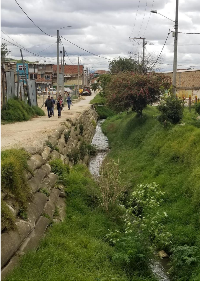
Fig. 11. Self-built intervention along the Limas Creek.
