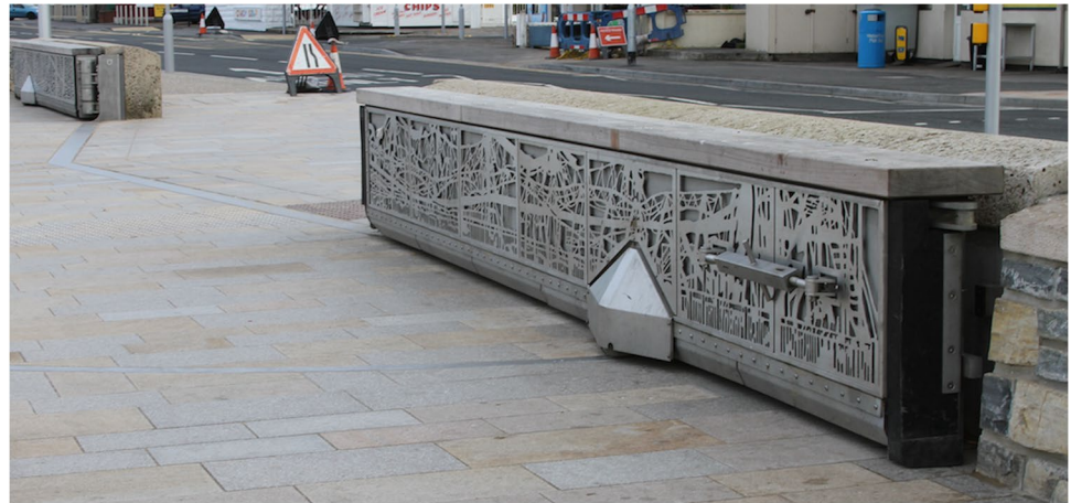
Fig. 4 One of the twelve flood gates on the esplanade's second, storm surge, 'splash wall' with part of a shopping area opening behind. This is the double gate outside the Grand Pier, the gate's pivot is in the centre (Fig. 2). Photo: ©W.B. Whalley, 2022 CC BY-SA 4.0
