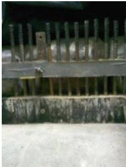
(c) Casting mortar on top of self-amalgamating tape at one end
