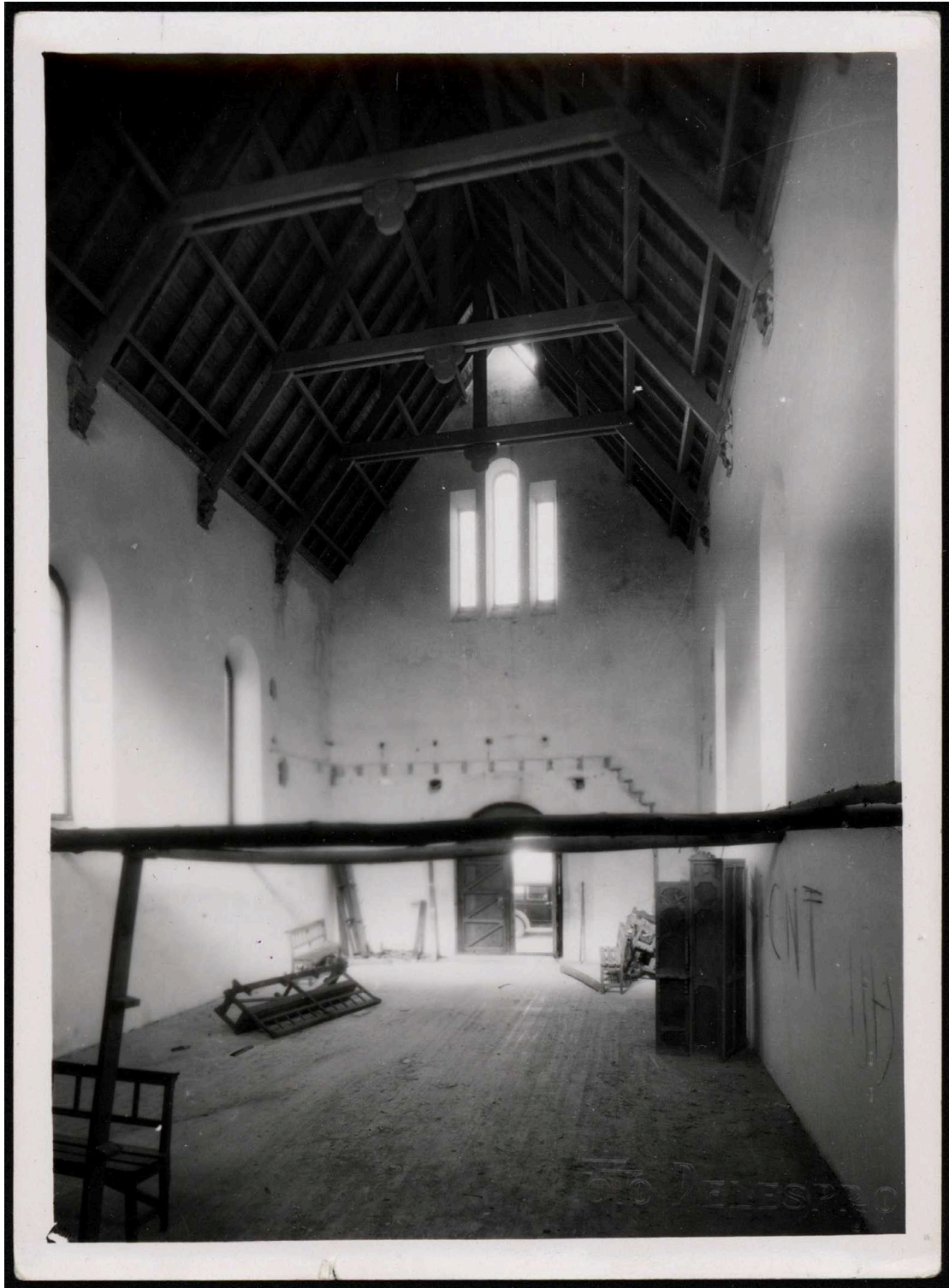
Figure 8: Capilla del Carmen, Suances (Santander) used by local fisherfolk to repair nets
