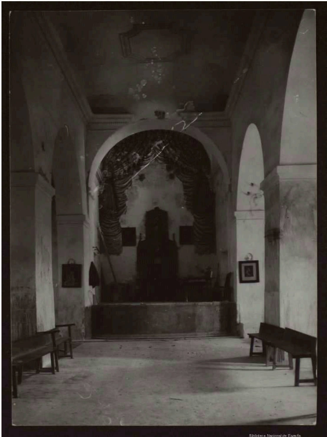
Figure 5: parish church of Yeles (Toledo) transformed into a theatre
