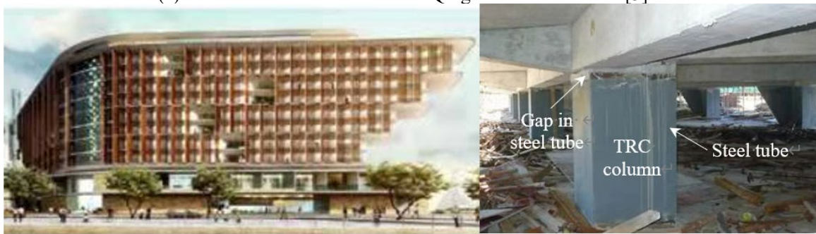
(b) Rectangular TRC columns used in China Resources Xiaojing Bay Hotel Fig. 1. Typical applications of TRC columns in engineering practices.
