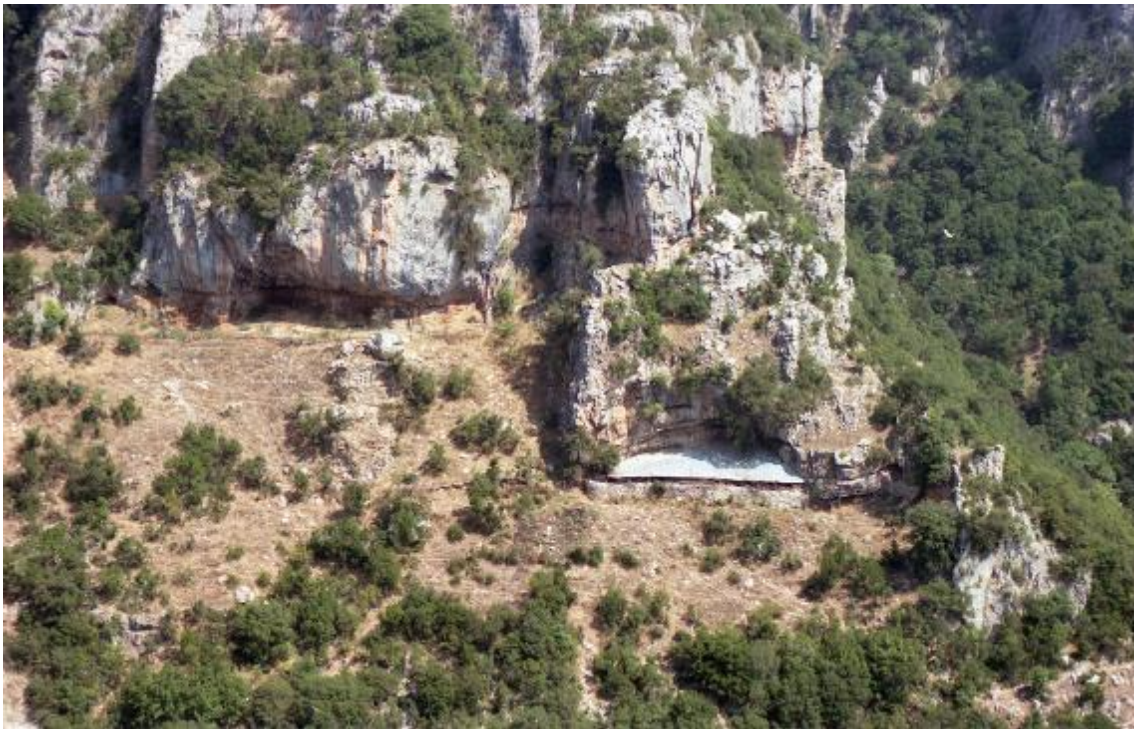
Figure 5 General view of the new goat shelter built into the cliff face high above Klithí.
