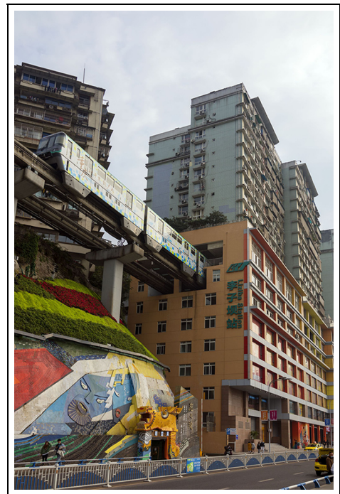
Figure 2. Liziba Light Rail Station in the sixth–eighth storeys of a residential high-rise.
