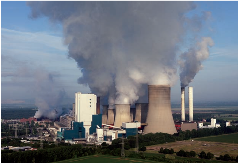
Fig. 2.9.3. The Niederaussem brown-coal power plant near Cologne, Germany. Coal-burning plants release carbon dioxide, fine particles, nitrogen oxide, and mercury, which can have a serious impact on public health. The coal ash produced by these plants contains contaminants such as arsenic, a known carcinogen.
