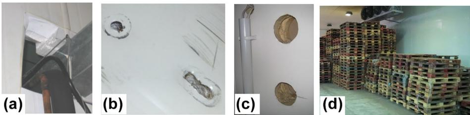
**Figure 1. Fire hazards observed by insurance inspectors: (a) damage around structural steelwork and pipe and cable installation; (b) forklift truck damage to ceiling panels; (c) holes through both sides of a panel, where pipework was going to be, or had previously been, installed; (d) typical accumulation of fire load in a sandwich panel building.**
