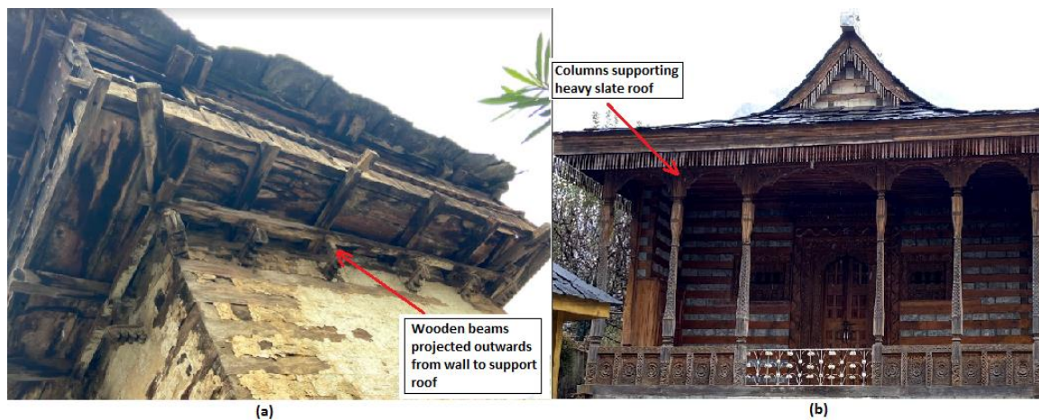
Fig 7: a Cantilevered balcony in old kath-kuni buildings, b Cantilevered balcony having columns to support slate roof.
