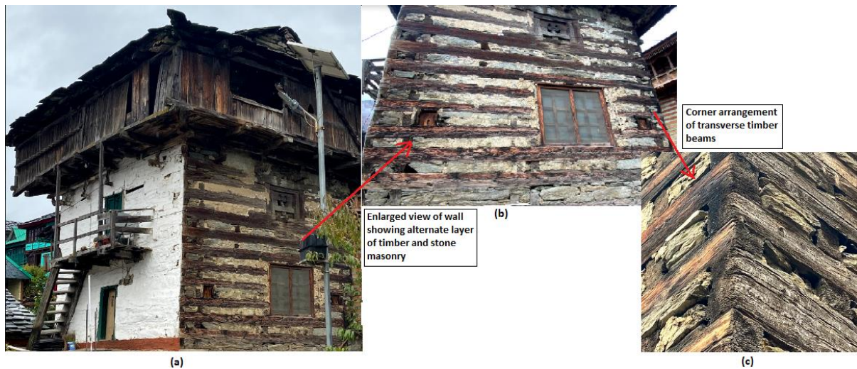
Fig 5: a Kath-kuni tower-like structure, b Enlarged view of Kath-kuni side wall c Corner details showing interlocking of transverse timber beams
