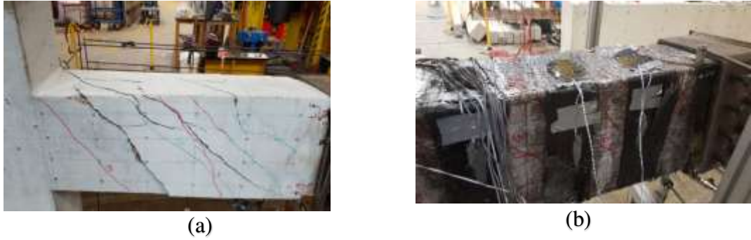
Figure 5. Beam cracks: (a) SH-U-C specimen, and (b) SH-S-C-H specimen
