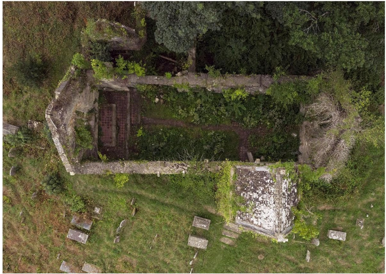
Figure 2. Top-down view: accessing the inaccessible, St Mary's Church, Tintern. © Isaac, 2019.
