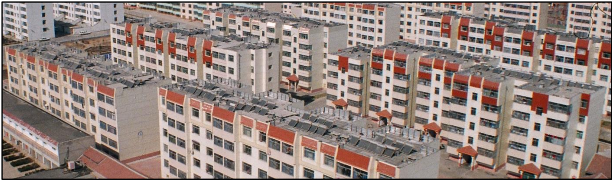
Fig. 1. A bird's eye view of the roof-mounted SWHs in Ju county, Rizhao. (Photo taken by Chengjun Ma, 1998)
