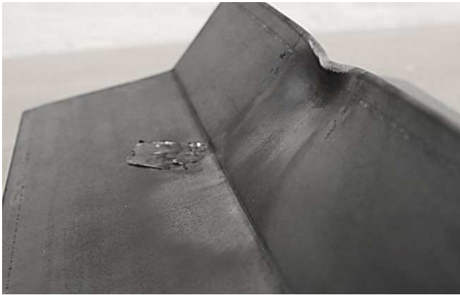
Figure 6 Photograph showing a blast tested double 150-75 V-structure (blasted side), tested at 50g. Source: Aashir Siddiqui/University of Cape Town
