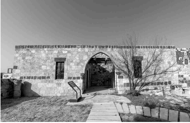
Figure 6. The courtyard houses in Ottoman Umm Qais were built using a mix of basalt and limestone salvaged from the remains of the ancient Roman city. This photo shows the Liwan House within the al- Husban courtyard house.
