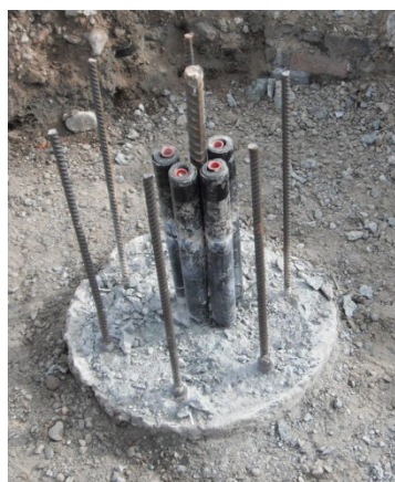
Figure 1. Example of a pile heat exchanger following pile trimming and prior to connection to the building base slab and the ground-source heat pump system. In this particular case the heat transfer pipes are centrally located and still retain their protective sleeves, which were used to avoid their damage during trimming.
