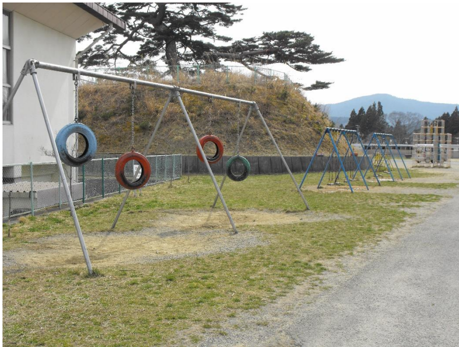
Figure 2: Reclaimed constructed space – part of a school playground in Minamisanriku, Miyagi Prefecture
