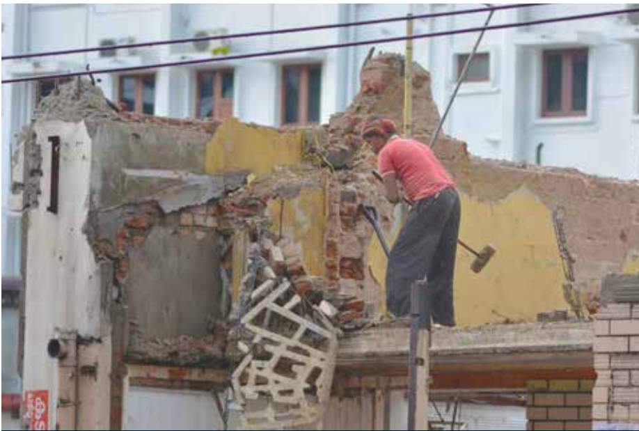
Manual demolition of a house in Mumbai, India; © rkl_foto (2015).
