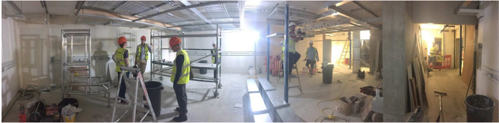
Fig. 29.19. The new laser laboratory at the University of Oxford under construction (image courtesy of the University of Oxford).
