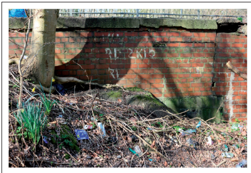
Figure 9. The brook passes under Barton Road Bridge and exits Kingsway Park to the west. Before culverting, this would have been a bridge over free-flowing water.
