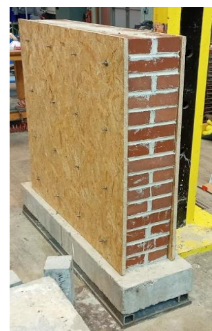
2-sided retrofitted wall
