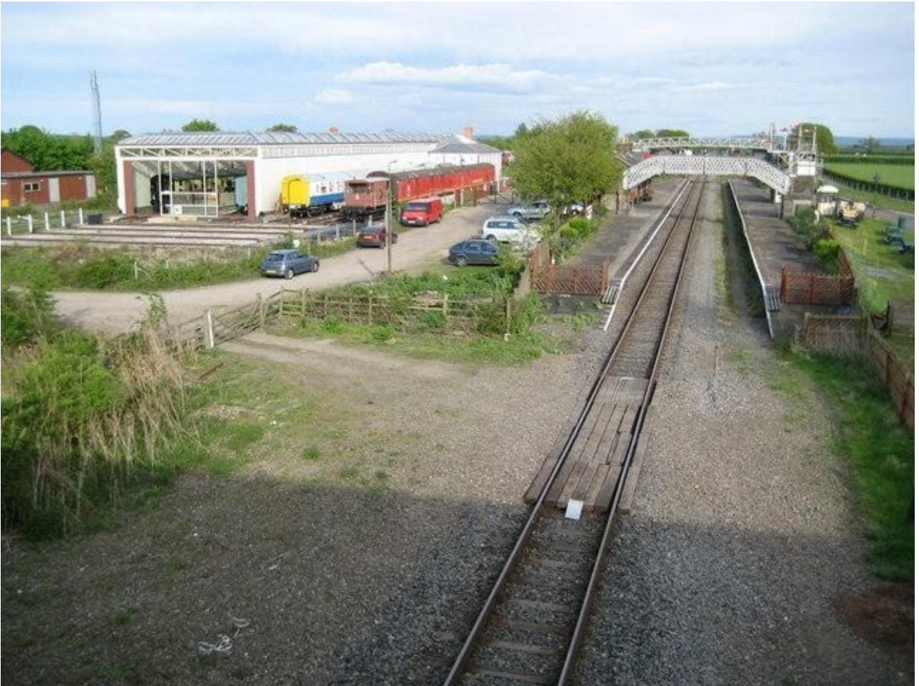
Figure 11: Quinton Road Station, the end of the line and subject of the closing scenes of Metro-land. This image was taken from the Geograph project collection. The copyright on this image is owned by Nigel Cox and is licensed for reuse under the Creative Commons Attribution-ShareAlike 2.0 license.
