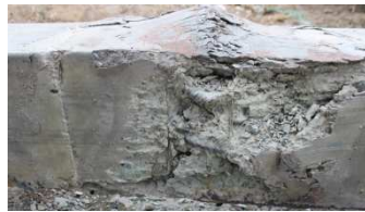
(e) Concrete crushing (TRC-0.6-0)
