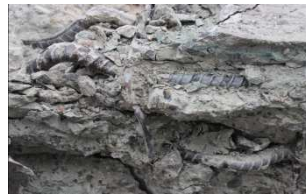
(f) Re-bar buckling (TRC-0.6-0)
