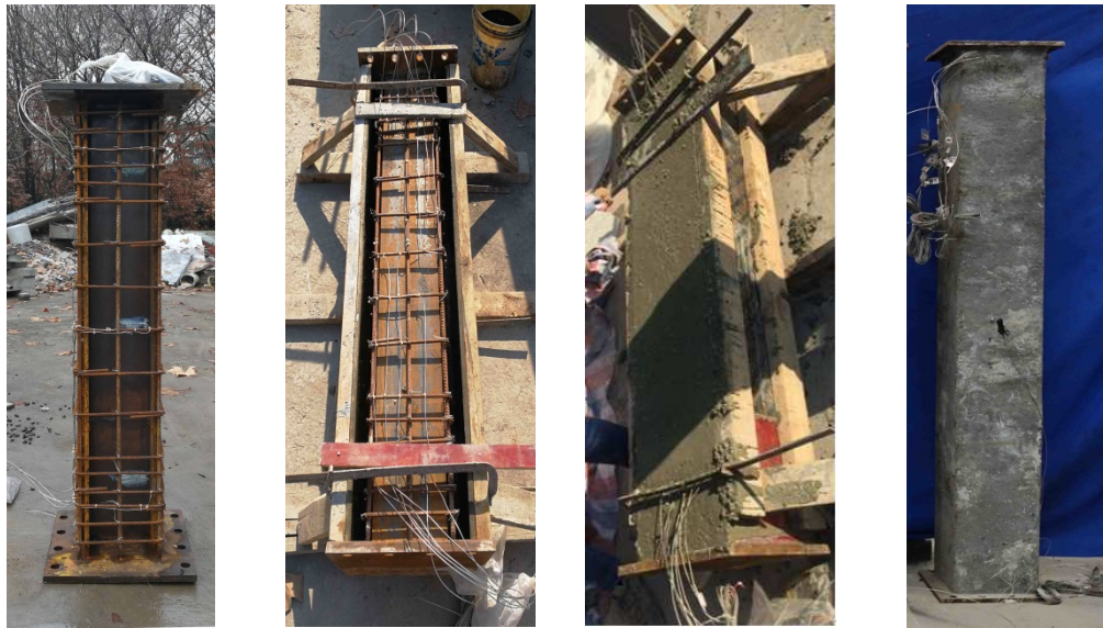
(a) Reinforcement cage installation (b) Formwork erection (c) Concrete casting (d) Specimen completion
