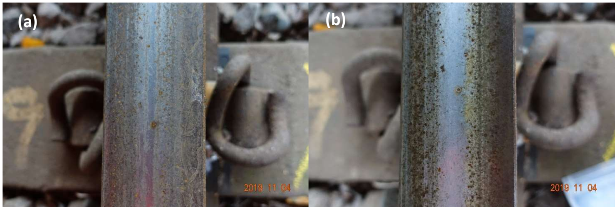
Figure 12: Contaminated untreated railhead (a), treated cleaned railhead (b)
