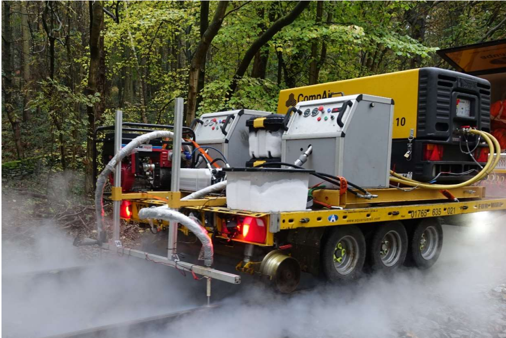
Figure 7. The RRV trailer mounted Cryogenic Cleaning Skid in operation
