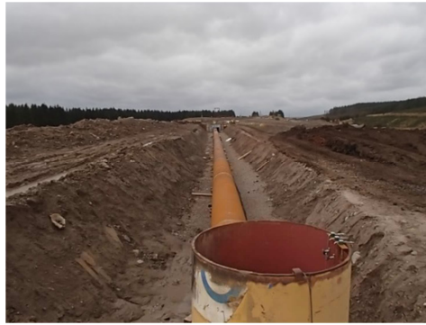
Fig. 1. Image of the test section prior to being backfilled.
