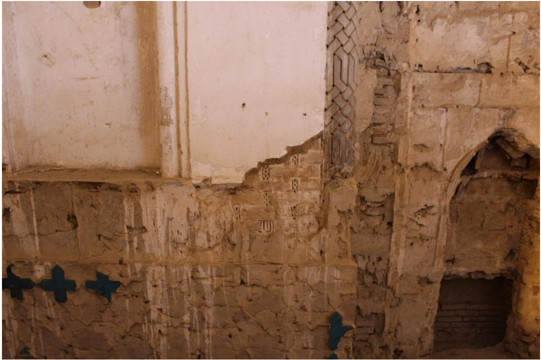
Figure 4: Rising joint mortar decoration beneath the (lost) band of lustre tiles, 'Abd al-Samad Shrine, Natanz
