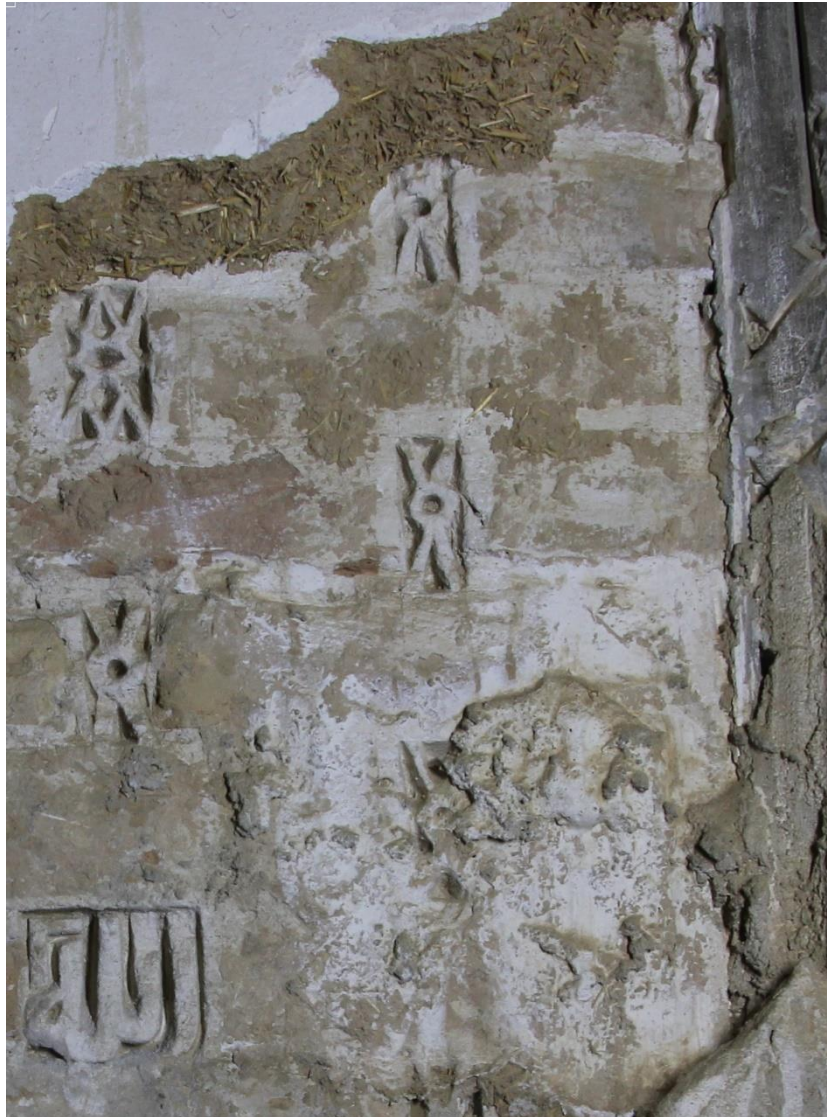
Figure 9: Rising joint plugs to the left of the mihrab, including ones extending underneath the stucco corner columns
