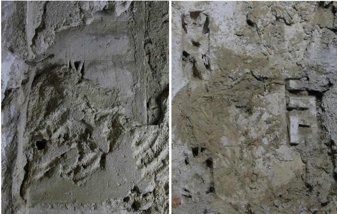
Figure 8: Incised construction lines in the earliest phase of brick decoration to the right of the mihrab niche (L), and square Kufic Allah brick plug (R)
