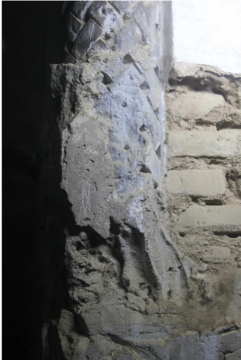
Figure 12: Base of the column to the right of the mihrab recess.
