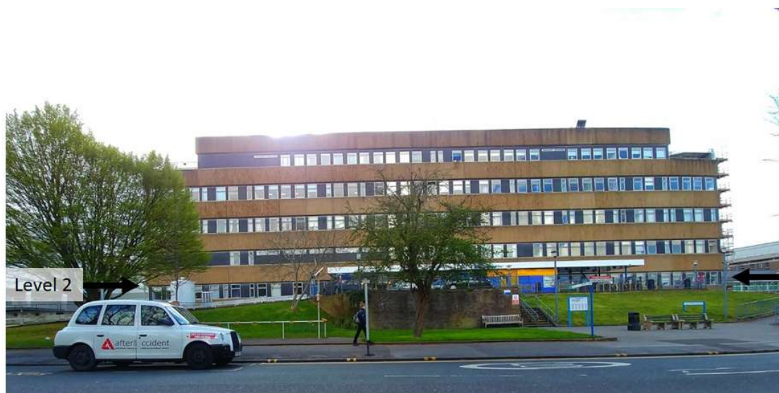
Figure 1. Photo of the Maternity and Gynaecology building taken from across the road. The black panels seen around the windows are asbestos. Level two is the ground floor of the building, highlighted by the black arrows, with the two entrances (Figure 2) located under the white awning.
