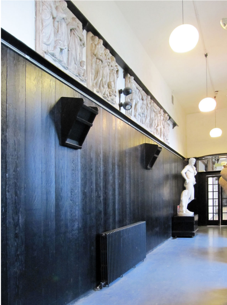
Figure 19. Hoppers for controlling ventilation in corridor.
