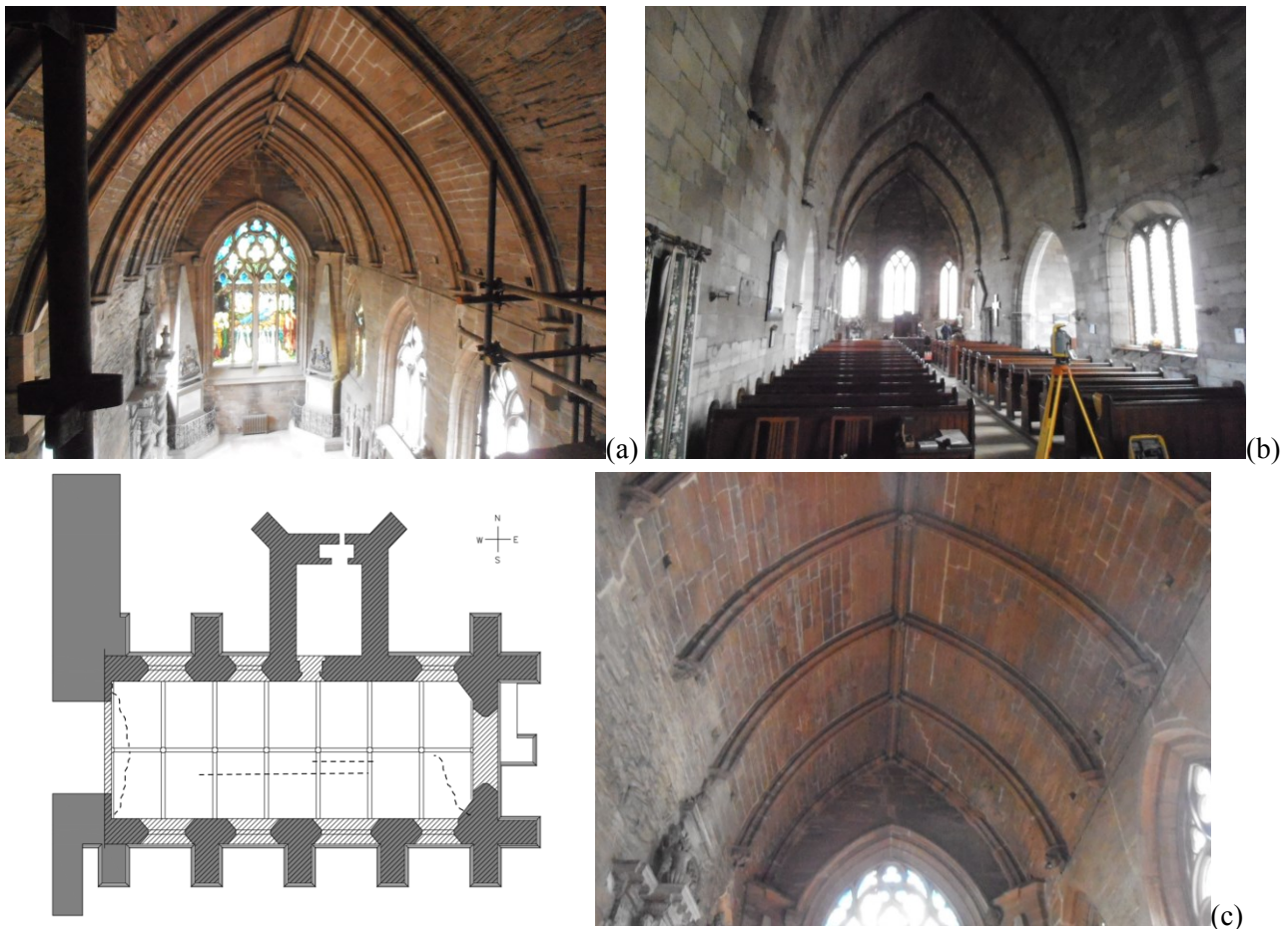
Fig. 1 – The earliest (a) (Bothwell 1398) and latest (b) (Ladykirk 1500) examples of barrel vaults in late-medieval Scotland churches. Crack pattern in Bothwell (c) due to deformation in the South wall from [27] and its appearance at the East end of the interior (following repairs in 2016), (settlement caused at the right-hand corner).
