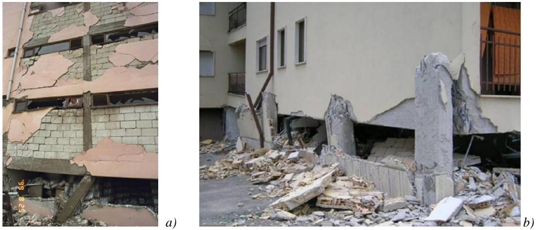
Figure 1. Effect of geometrical irregularities in distribution of infills: a) Adapazari-Turkey (1999); b) L'Aquila-Italy (2009).
