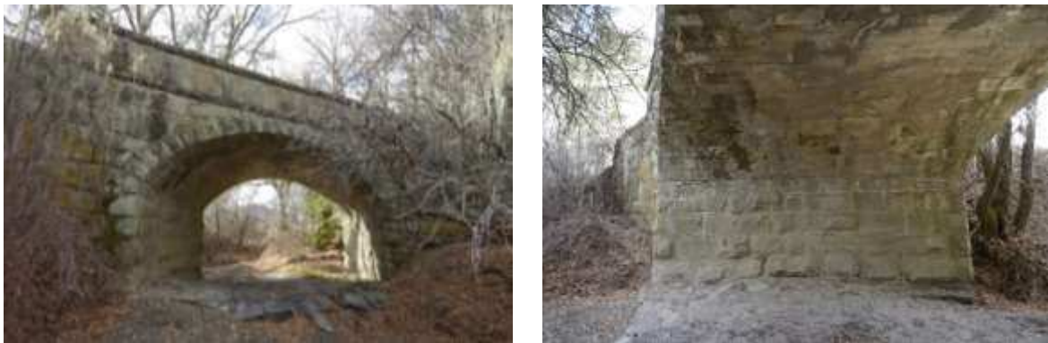
(a) False skew arch: Maxwell Creek Bridge, Napa County, California, USA (courtesy of Mark Yashinsky)
