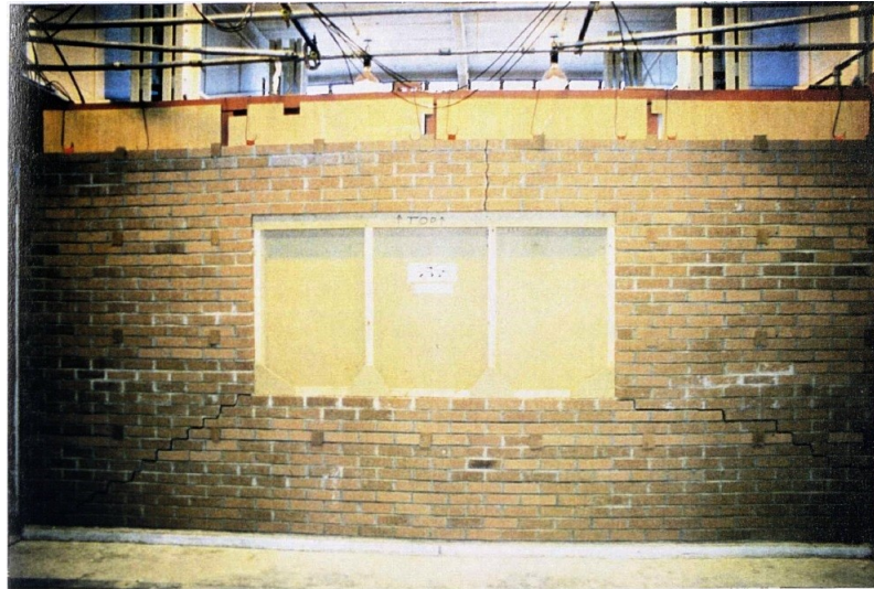
Figure 10: Crack patterns in the experimental study (SB02)
