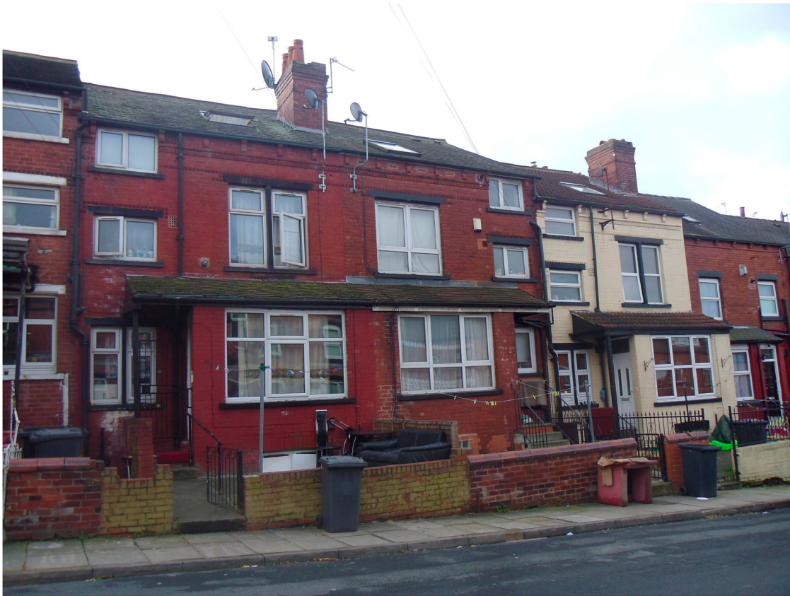
FIG. 12. Split level back-to-backs in Luxor Avenue. One side of the house has full-height floor levels, while the other side has lower floor to ceiling heights to create extra space in the small attic bedroom.
