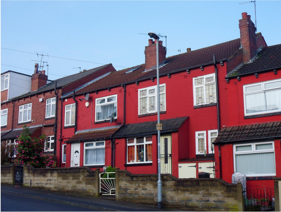
FIG. 11. Small, cottage-style back-to-backs in Arley Street. These did not have attic rooms or basements.
