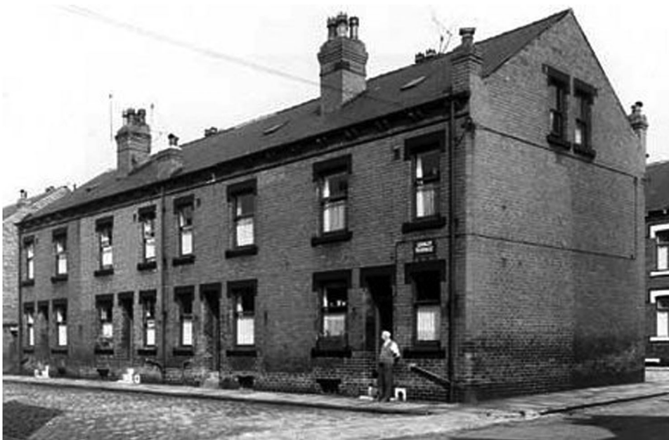
FIG. 5. Stanley Terrace was built in 1890. The chimneys positioned to the front of the property indicate that the copper was positioned in the scullery. Image: By kind permission of Leeds Library and Information Services, www.leodis.net
