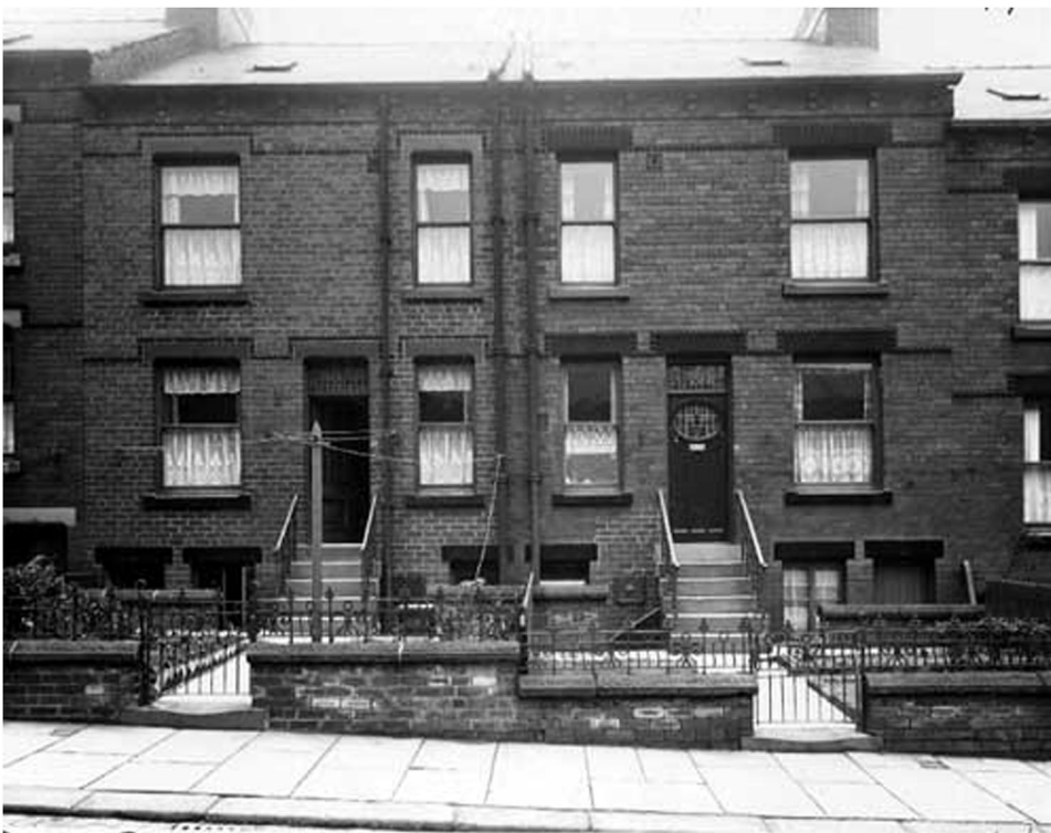
FIG. 8. Superior back-to-backs in Darfield Place, Leeds. The presence of gardens allowed the ground-floor level to be raised and accessed via steps, which had the benefit of positioning the basement at semi-subterranean level. Image: By kind permission of Leeds Library and Information Services, www.leodis.net
