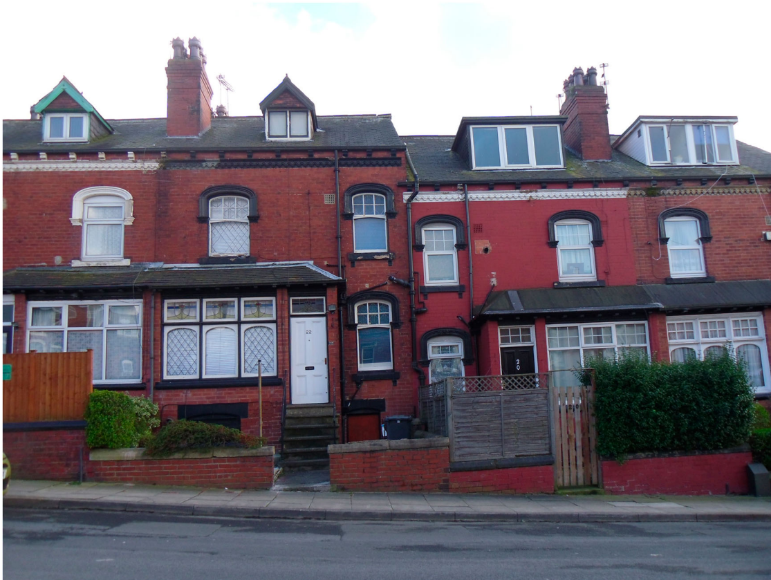
FIG. 10. Luxor Avenue back-to-backs, built around 1907. These were particularly decorative, incorporating dormer and bay windows, the latest style of window design, stone window surrounds and a small entrance hall.
